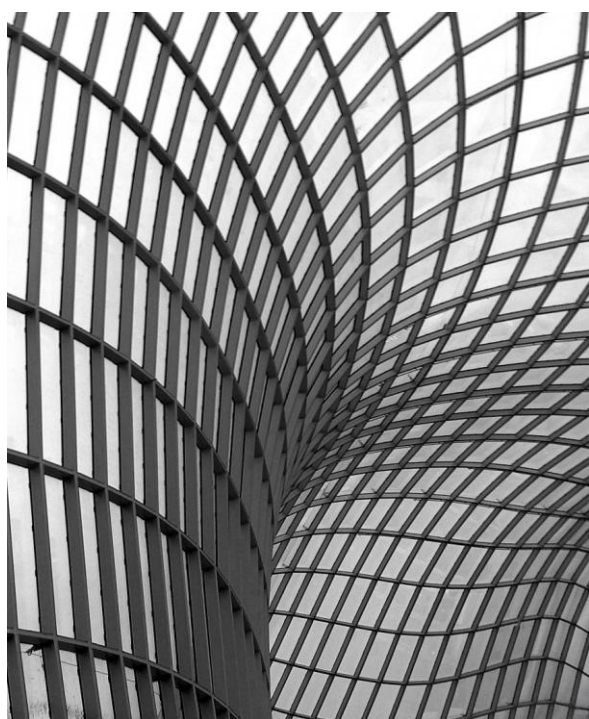
TIGHT SQUEEZE - ROOF at CHADSTONE SHOPPING CENTRE – Felix Menke
